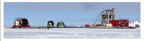
• With hot water and a special drill. It is much easier than evacuating a cavity deep in the earth
